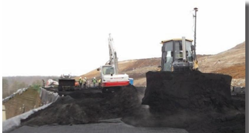
Construction of an eMSE berm using coal combustion residuals with geogrid reinforcement.
