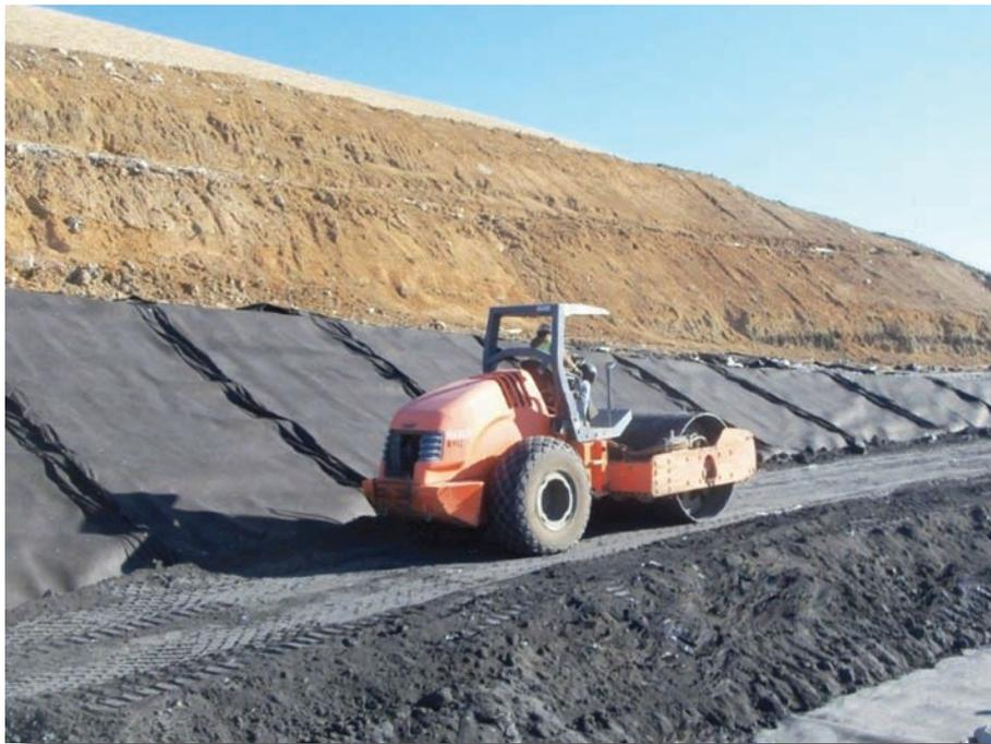
Figure 2: eMSE berm construction using CCR and impacted soils as fill material.
